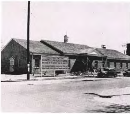
Tent 22, Oklahoma City, Okla., is now constructing the Health Center, to provide free housing for the Salvation Army Health Clinic and Tuberculosis Clinic, and Maternal Health Center Clinic.
